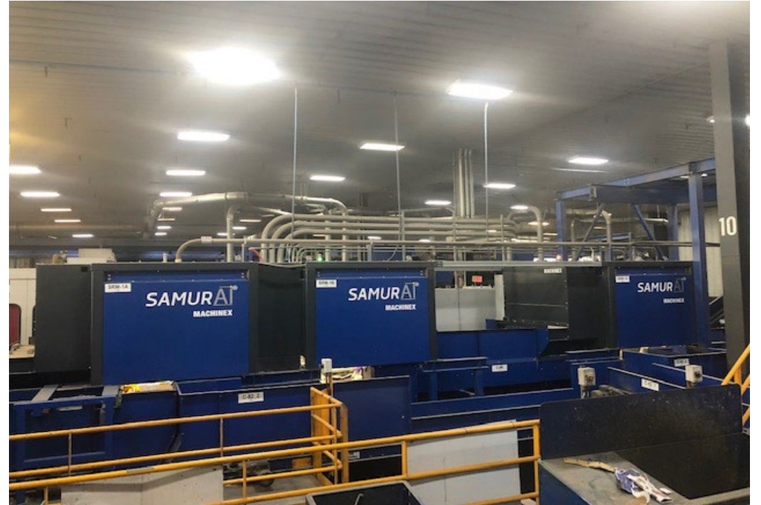
Rumpke PP robot installation- The Recycling Partnership PP Grant- 2021
